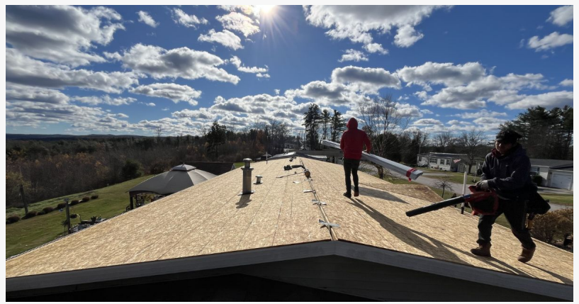
The Paramount Roofing NH crew at work on a full roof replacement in New Hampshire.
