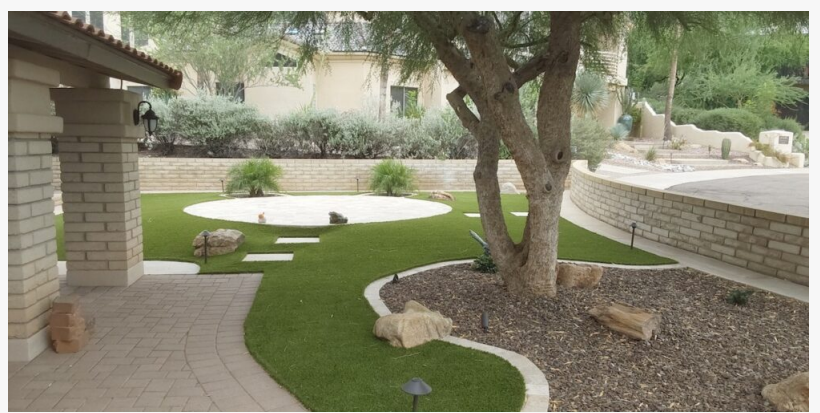
Artificial Turf Installation Phoenix
