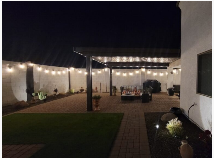
Landscape Lighting Installation
