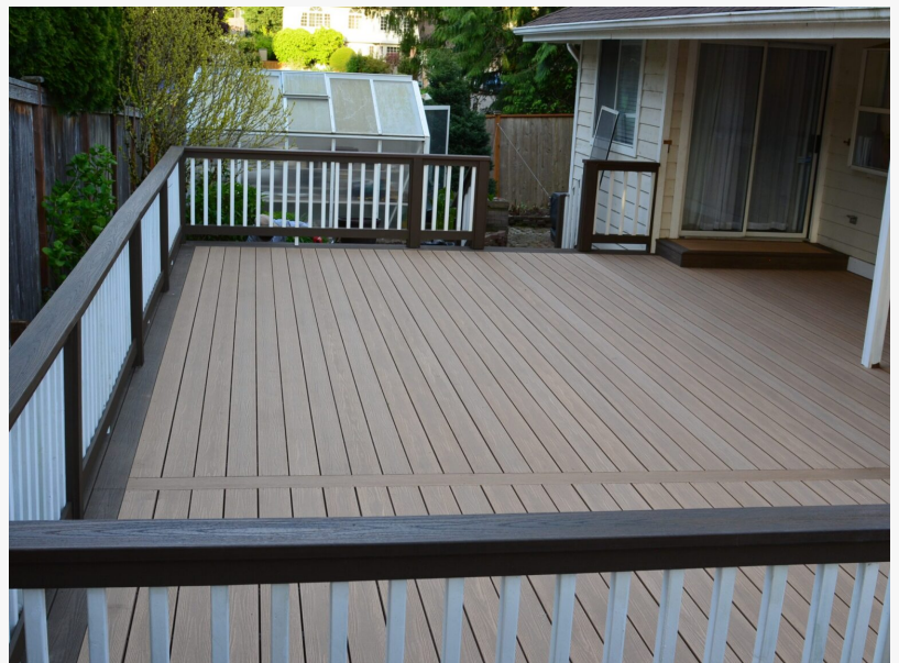
Deck and Patio Installation
