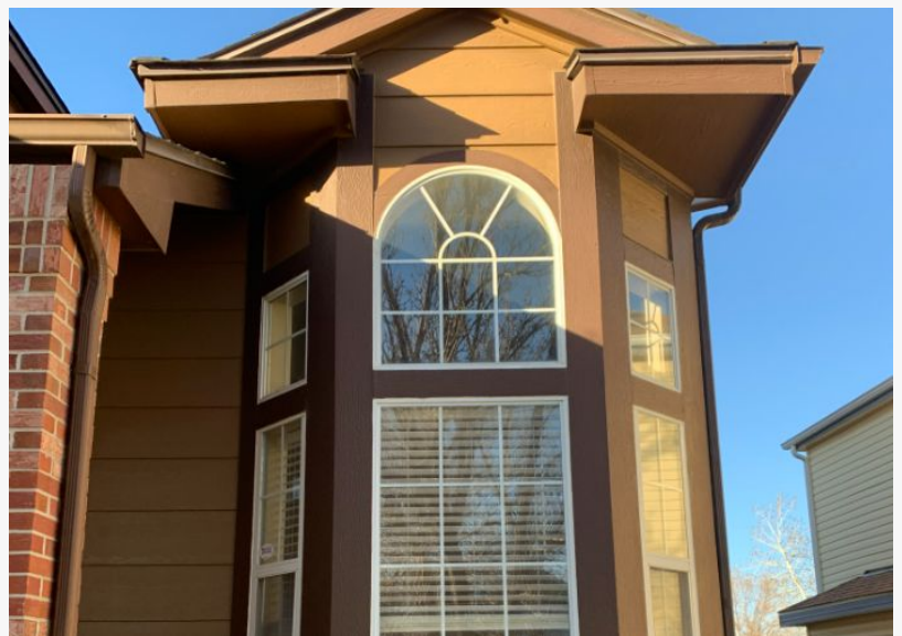
Project for new customer window replacement installed by Conservation Construction
