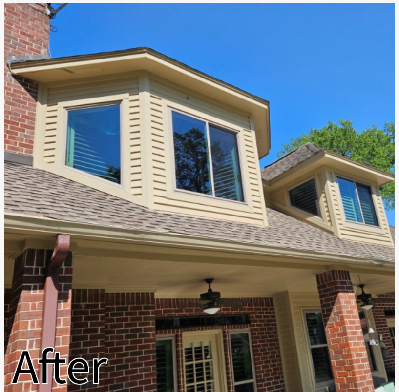
After window replacement project for a Denver home
