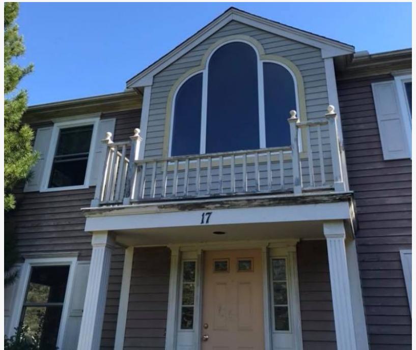
Custom window replacement for a Rhode Island home
