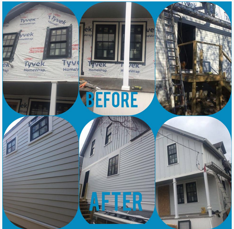
Before and afters of United Better Homes siding installation projects
