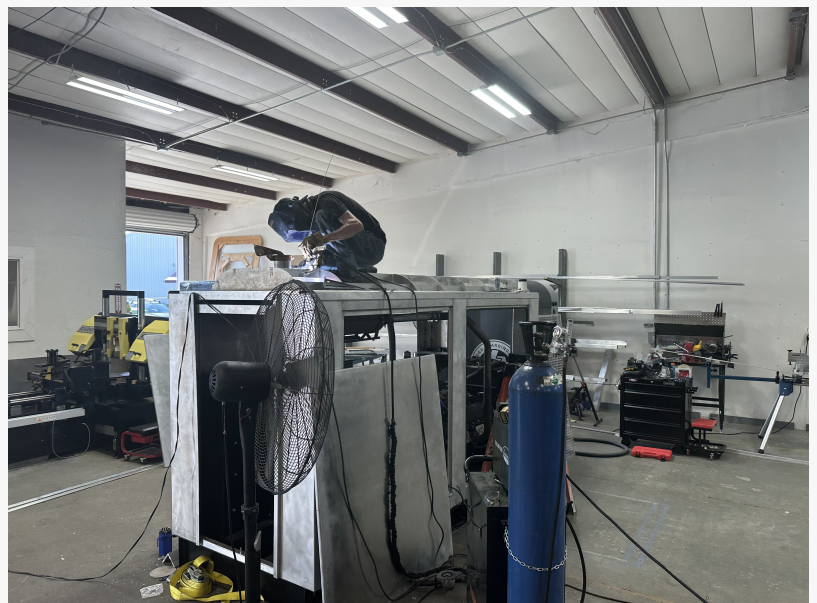
Custom Mobile Charger Buildout
