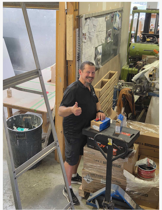
Electrified Marina lead technician Robert Rubano about to install batteries on Wada Hoppah
