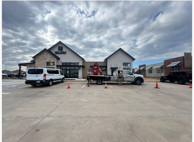
Our Team at site, finalizing the work.
