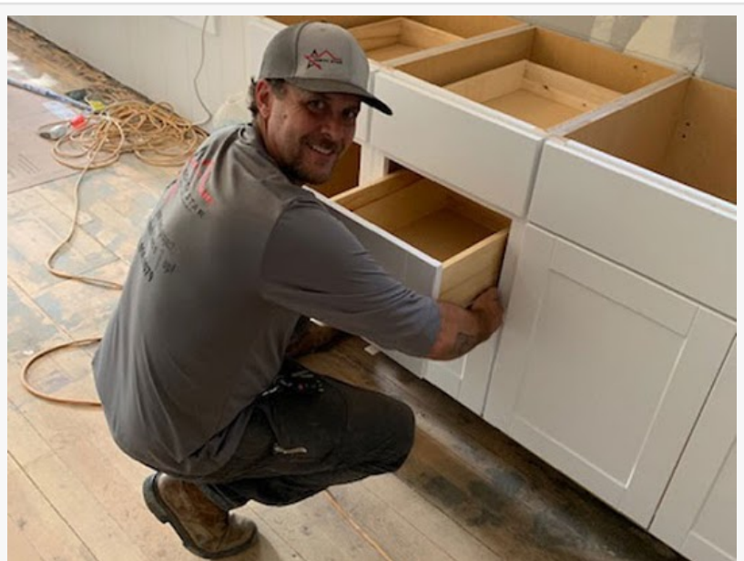
North Star contractor completes a kitchen remodel project in Boise
