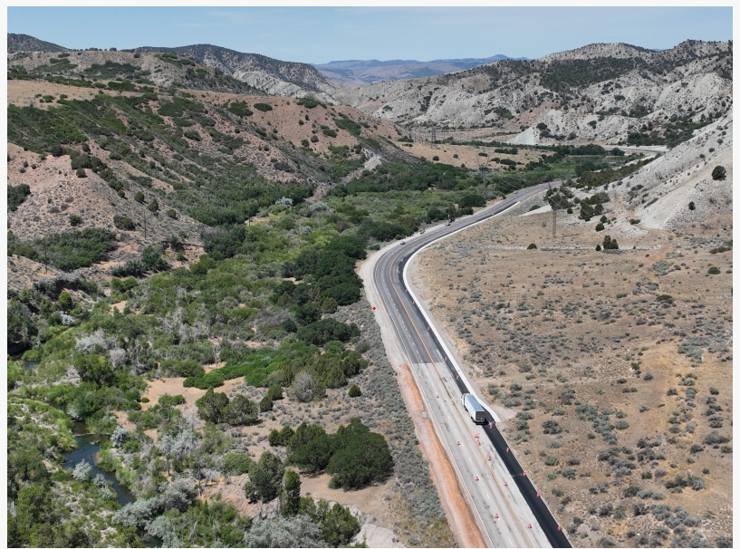
SR-132 improvements from milepost 38.1 to Nebo Loop Road, a UDOT passing lane and intersection project on one of Utah's scenic byways, currently in construction.
