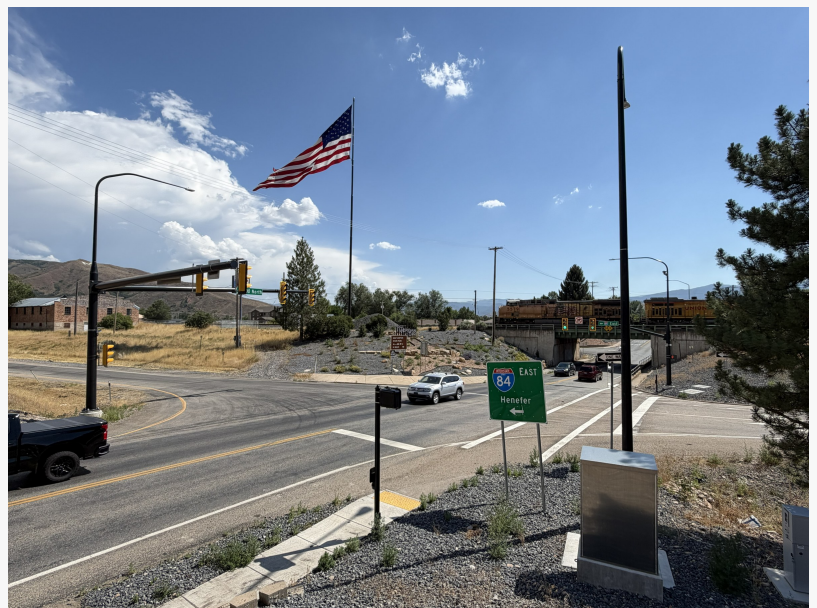
SR-66 (300 North) at the I-84 eastbound ramps in Morgan, Utah. O'Neill & Company designed Morgan's first traffic signal, improving safety and operations at a critical freeway interchange.
