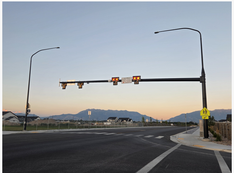
Pedestrian hybrid beacon at SR-193 and 4375 West in West Point, Utah, one of more than 100 pedestrian safety improvements O'Neill & Company has designed statewide.
