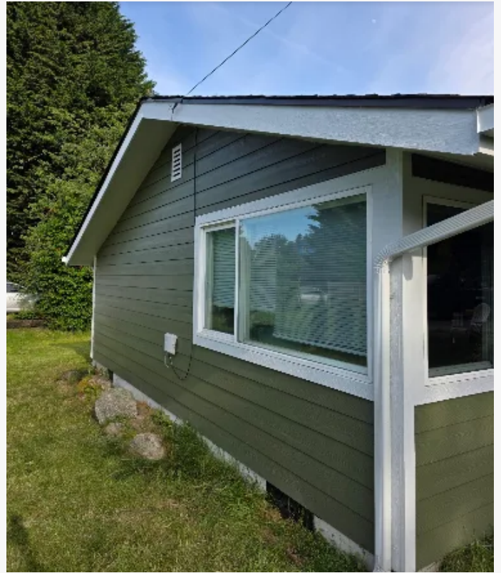
Completed siding and trim installation project showcasing quality craftsmanship by Final Touch Construction LLC.
