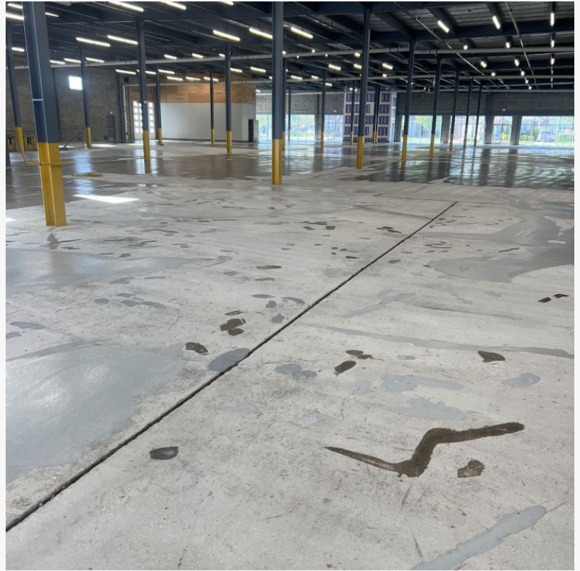
Substrate Repair Prior To Application
