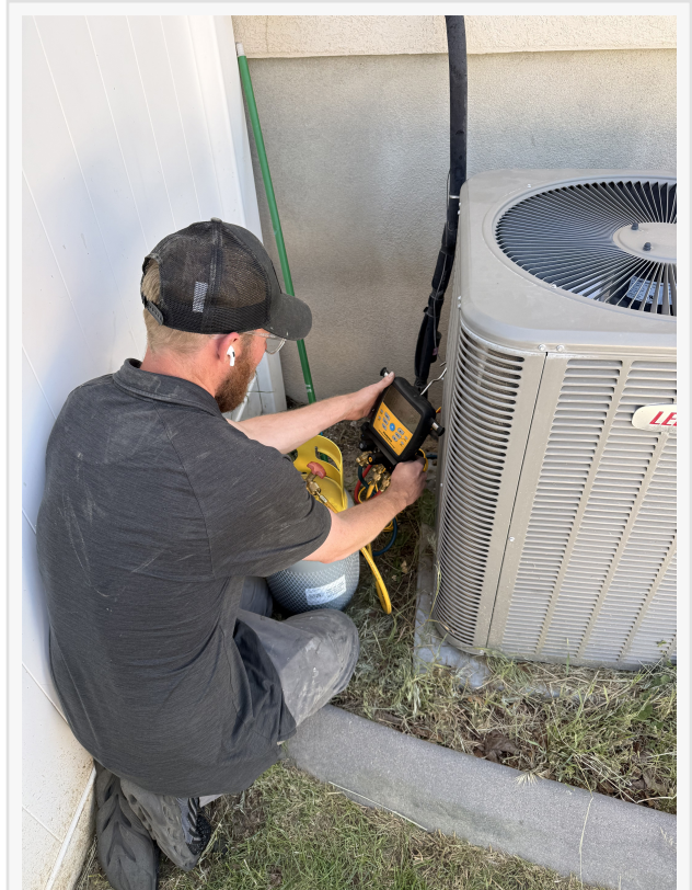
Prompt and professional AC repair in West Jordan, featuring a technician performing a comprehensive system diagnostic and refrigerant check to restore home cooling performance.
