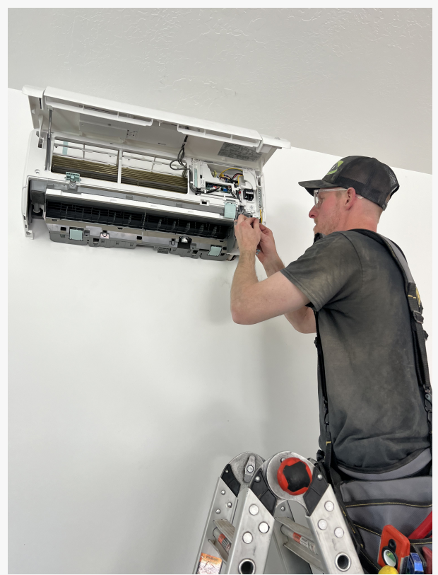
An expert HVAC technician performing a wall-mounted ductless mini-split installation and AC repair in West Jordan to ensure optimal indoor climate control.
