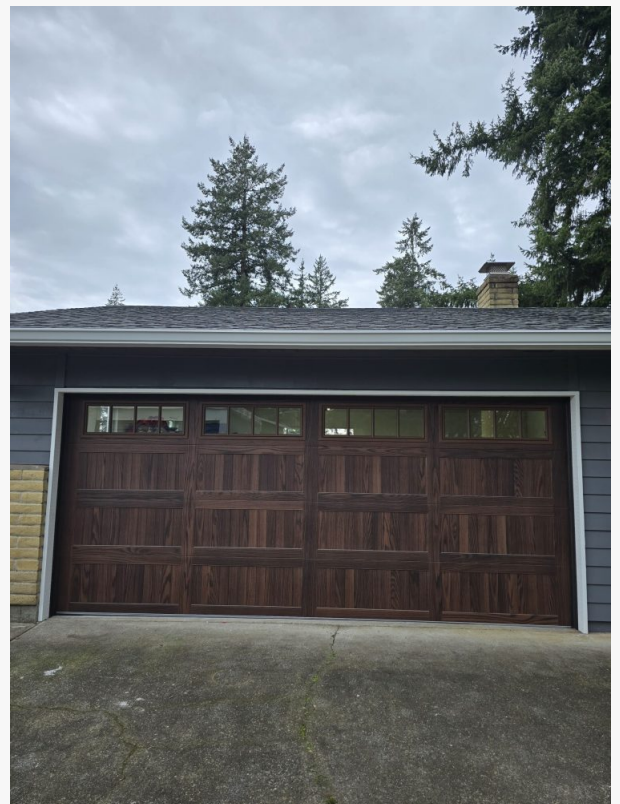
Garage Door Built
