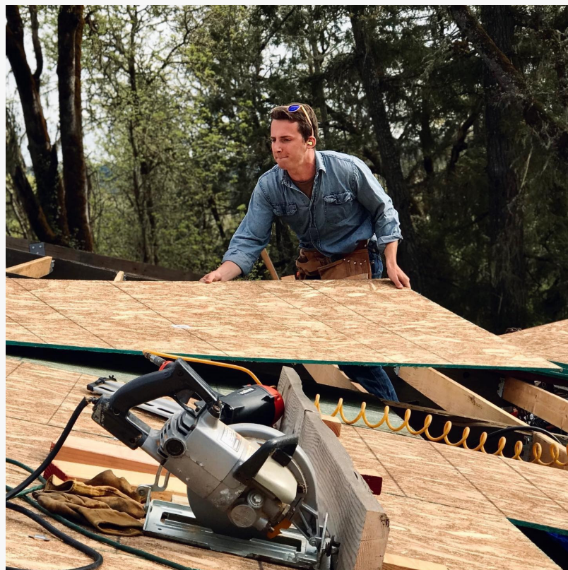
Aaron Cherry on site during roof framing and sheathing on a Roseburg property. Cherry stays involved with projects from the initial evaluation through completion, coordinating roofing companies, electricians, plumbers, excavation contractors, septic speci
