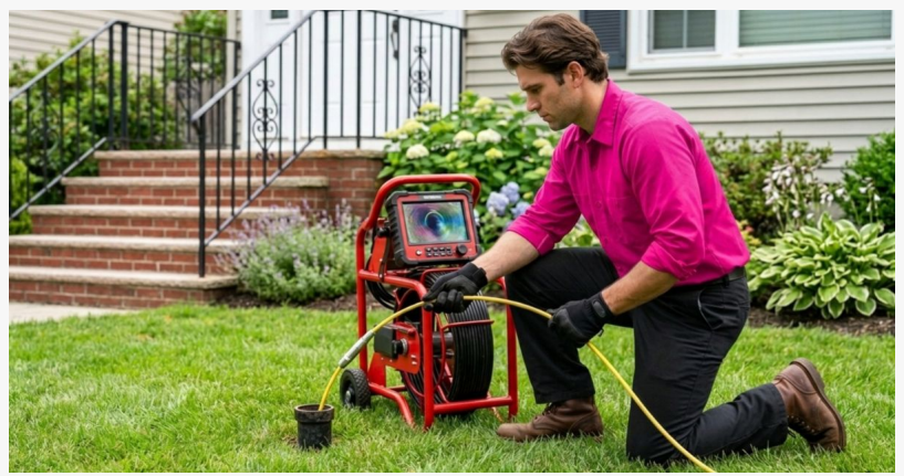
A Pro Trenchless Services technician using specialized inspection equipment to evaluate underground sewer pipes and provide efficient trenchless solutions.
