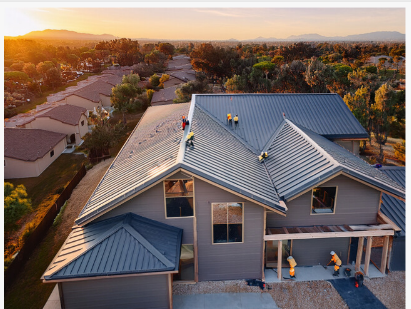
Family Roofing - New Roof Installation
