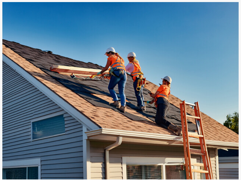
Family Roofing - Roof Repair
