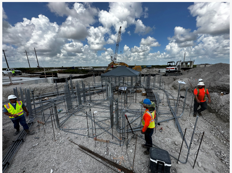
Electricians working at Central Everglades Planning Project (CEPP)
