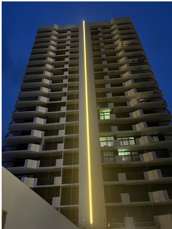
Old Port Cove Architectural Lighting Project 185-foot outdoor LED strip lighting systems
