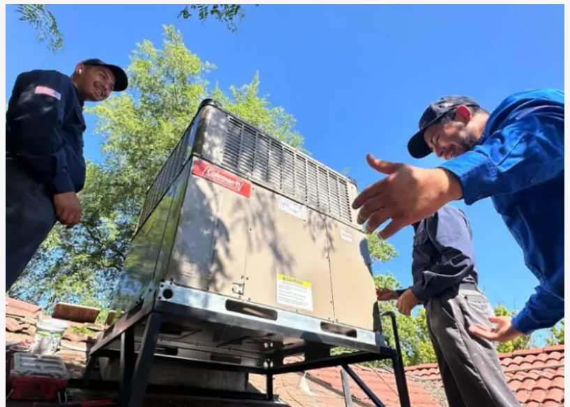
Mechanical Air LLC technicians performing professional installation and maintenance on a commercial rooftop HVAC unit.
