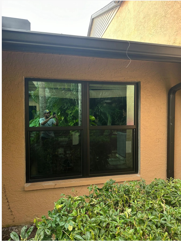
Hurricane-Rated iMPACT Windows Installed by Local Experts
