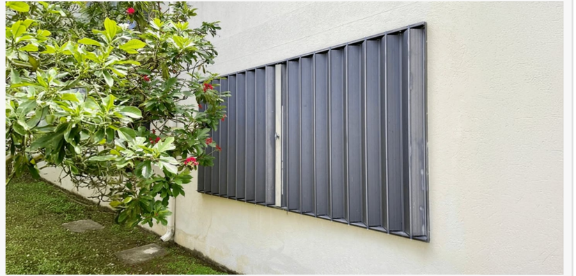
Dependable Hurricane Shutters Installed By Florida Experts
