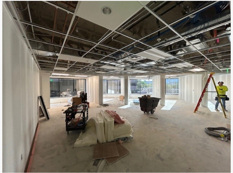
Pictured: Commonwealth Land Title Phoenix NCS' office mid-construction during expansion phase
