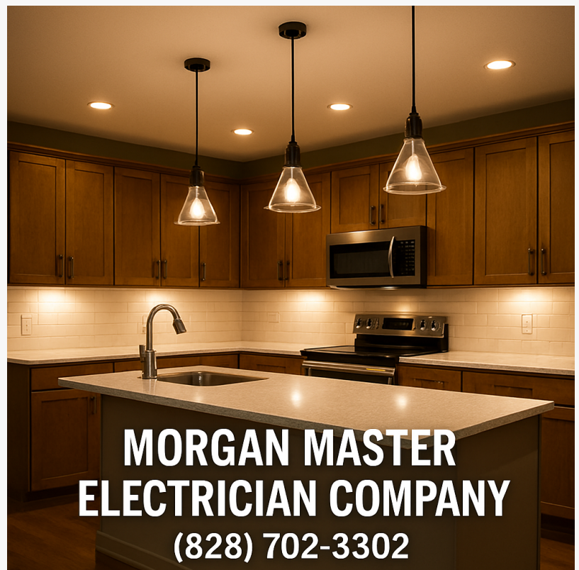
Kitchen Lighting Installation
