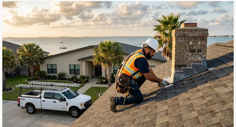
Roof Repair in Portland, TX
