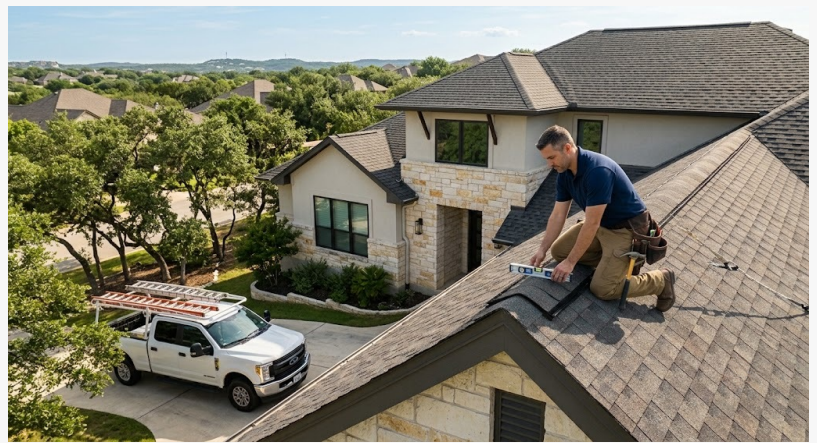
Roof Repair in San Antonio, TX
