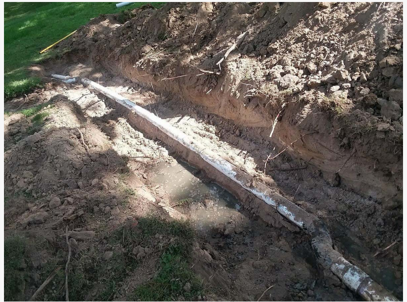
Out with the old plumbing, in with the new!
