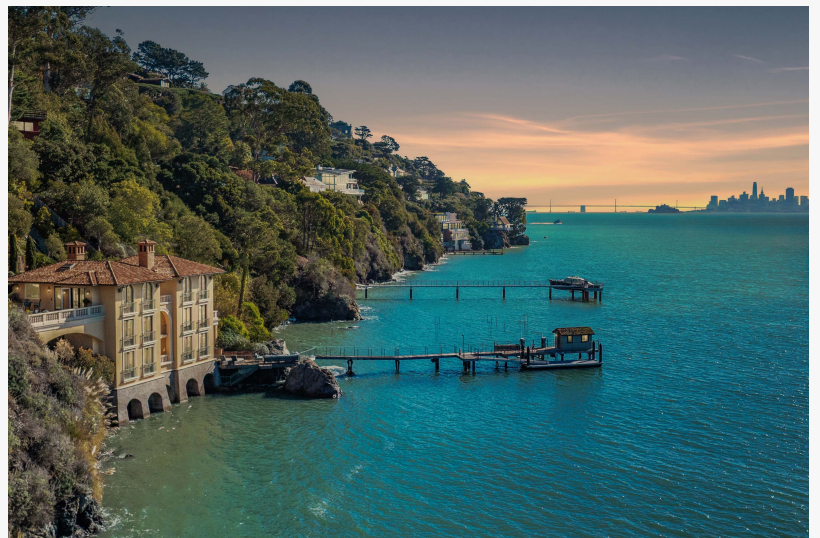
Designed by Andrew Skurman, Built by Red Horse Constructors
