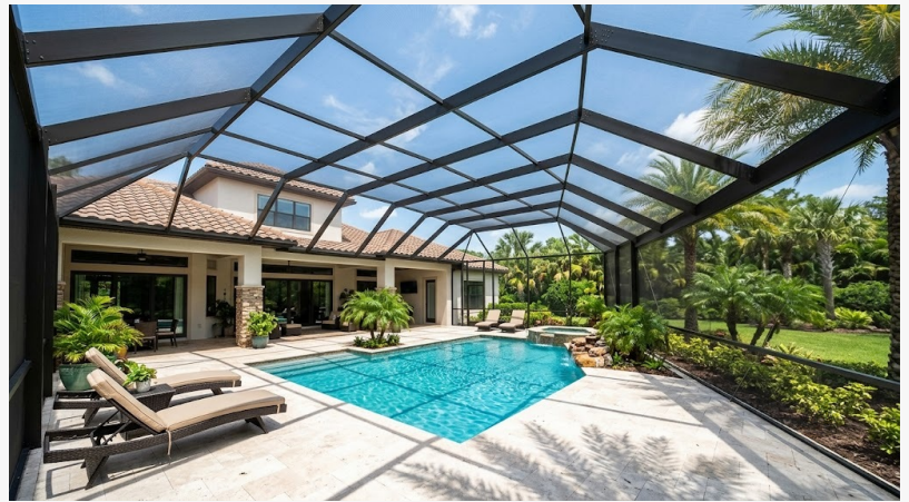
Pool Screen Enclosure in Winter Park, FL
