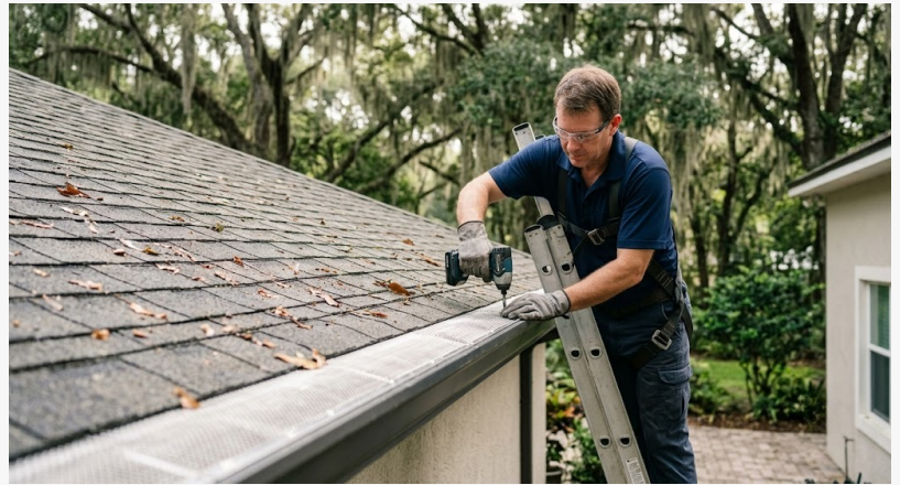
Gutter Guard Installation in High Springs, FL
