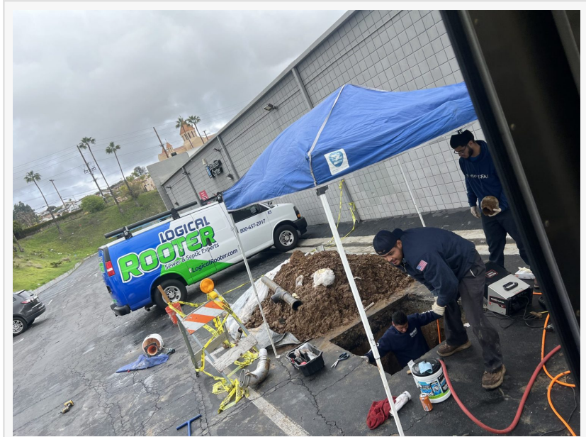
Logical Rooter Drain Cleaning Team Replacing a Pipe in Los Angeles
