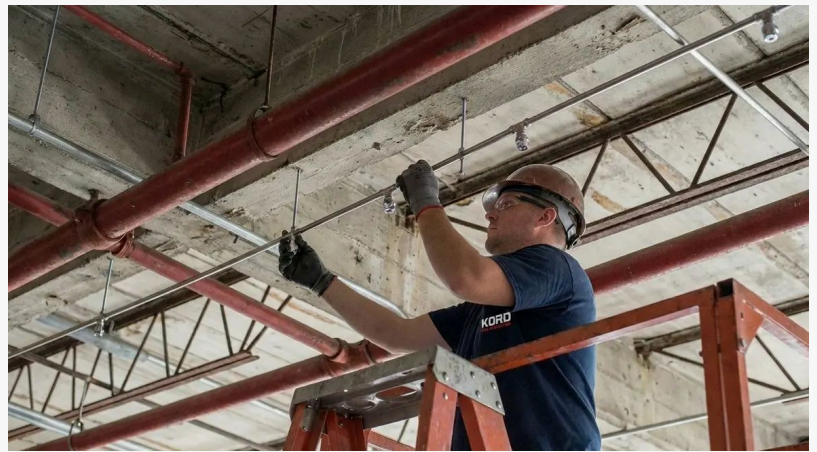
Fire Sprinkler Work
