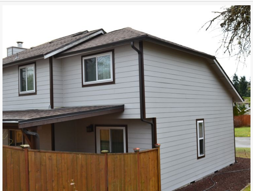
Expert-Residential-Siding-Installation Gab Construction
