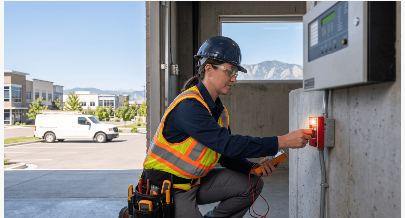
Broomfield Fire Alarm Monitoring
