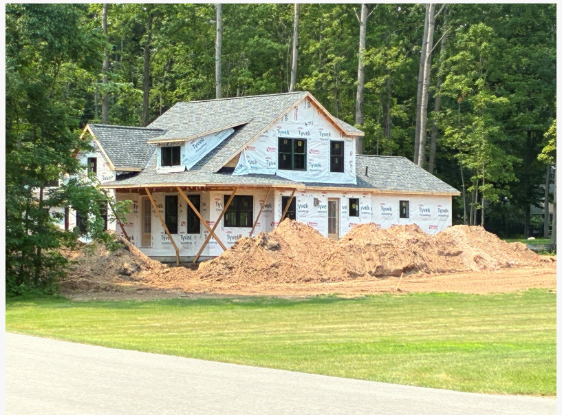
Home Building in Process on the Golf Course
