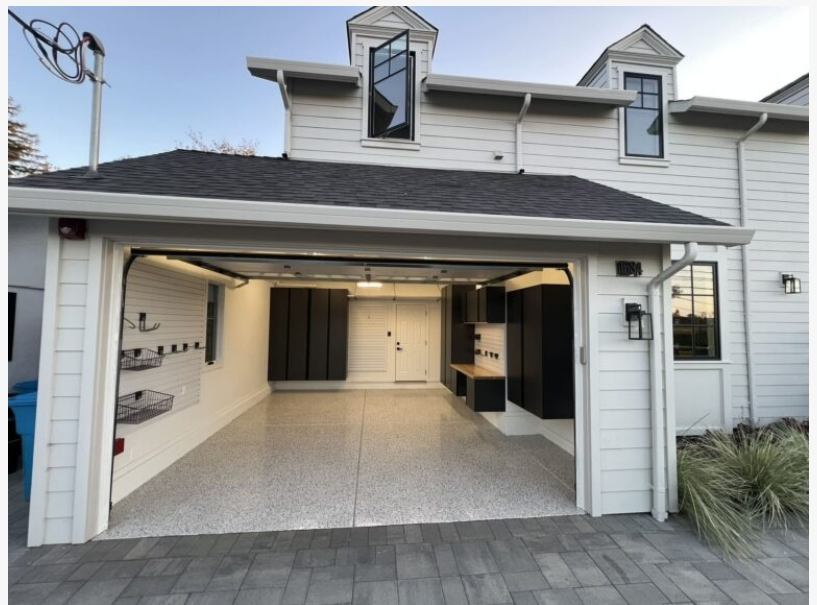
garage storage system Orinda CA
