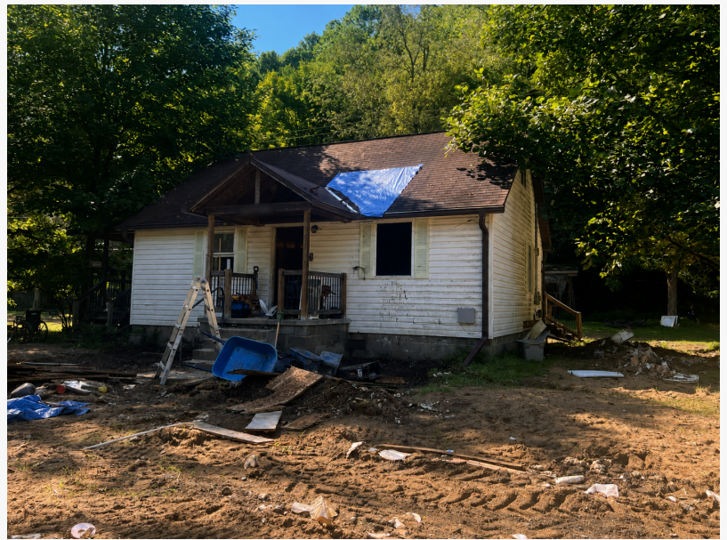
Flood damaged home in West Virginia
