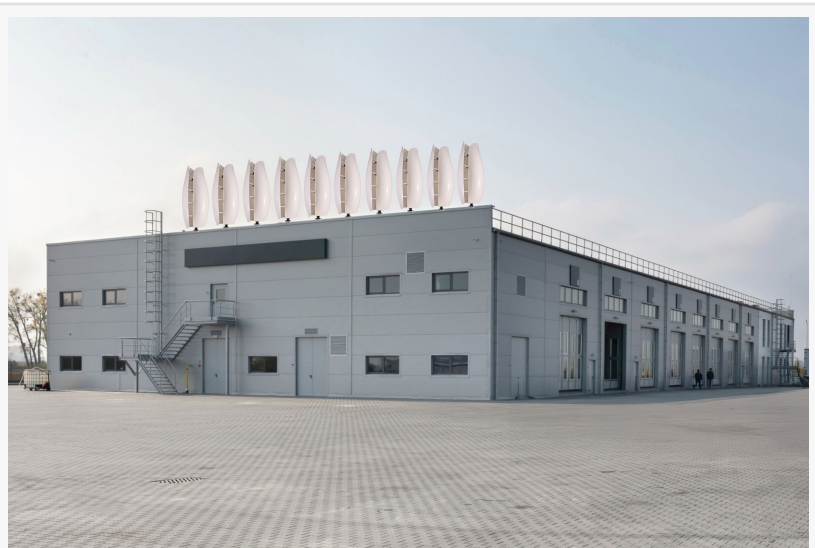
Row of wind turbines on roof
