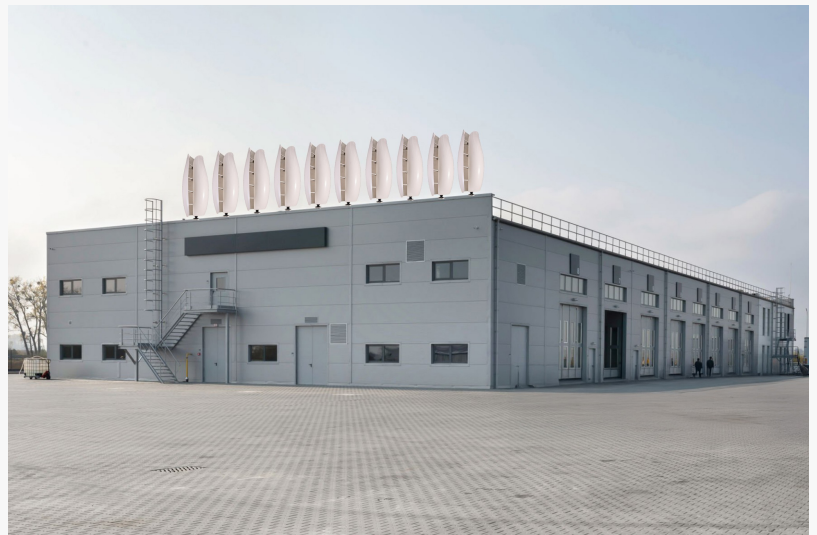
Row of wind turbines on roof
