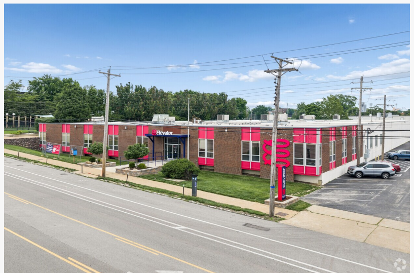
Elevator St. Louis Building Entrance
