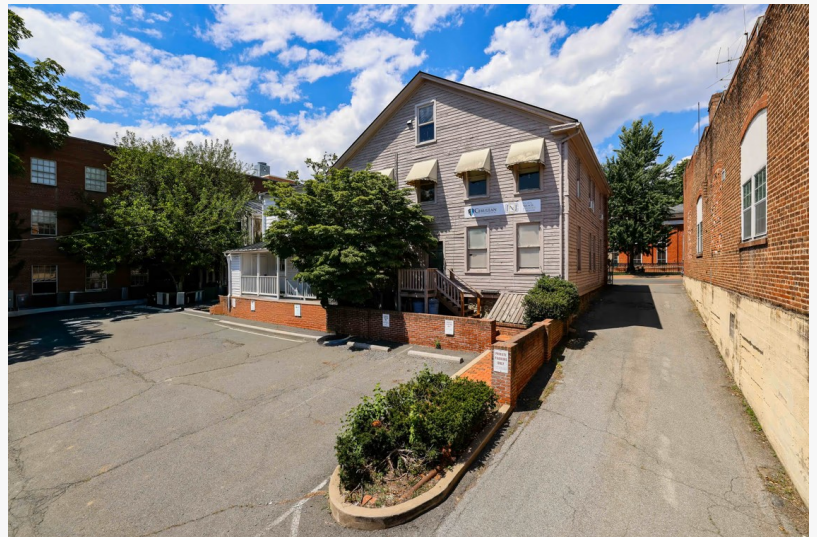
3, 5 & 7 E Market Street, Leesburg, VA 20176
