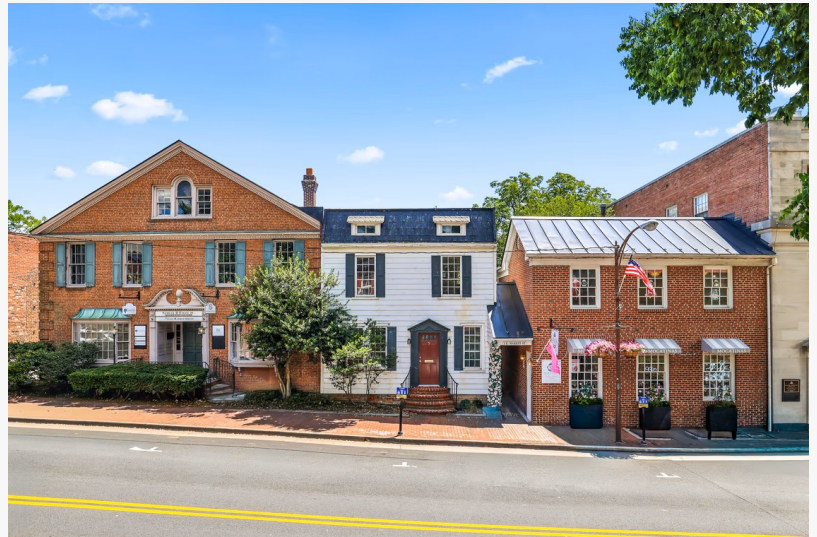
3, 5 & 7 E Market Street, Leesburg, VA 20176
