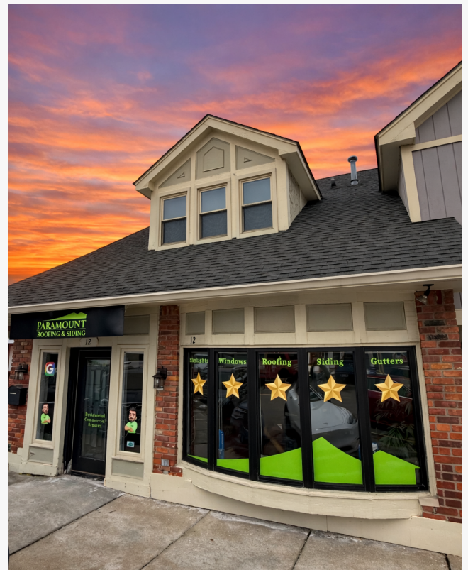
Paramount Roofing - Plymouth Location
