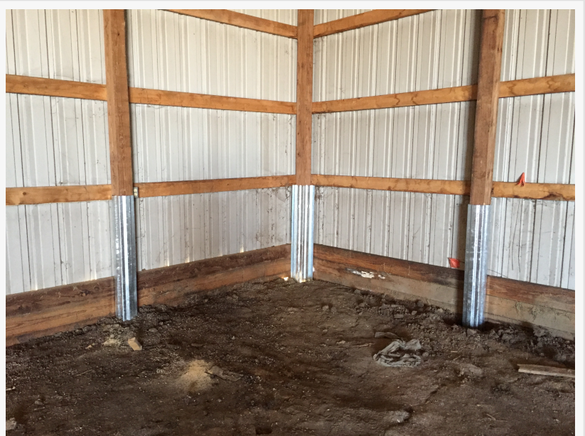
Anthem Built pole barn repair
