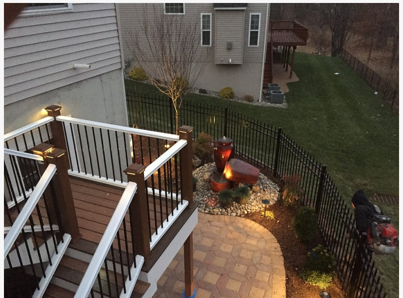
Fence and deck installation
