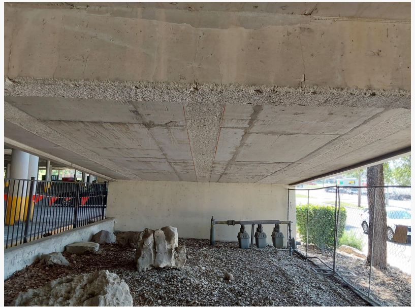
Parking deck repairs
