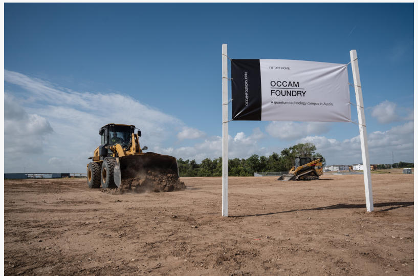
Earthwork underway at the Occam Foundry site in Austin, Texas, Aug. 14, 2026. The banner marks the future home of the quantum technology campus announced today by Texas Quantum Partners and Samara. (Chris Lake)
