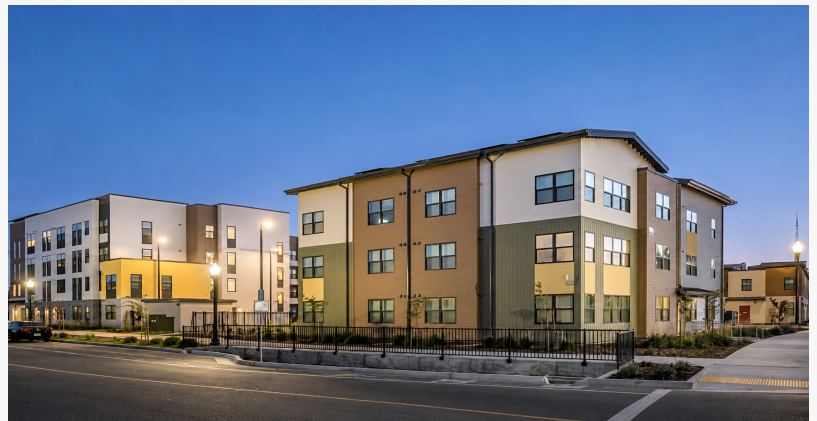
The dirt at the new Mirasol Village in Sacramento tested positive for chlordane.
