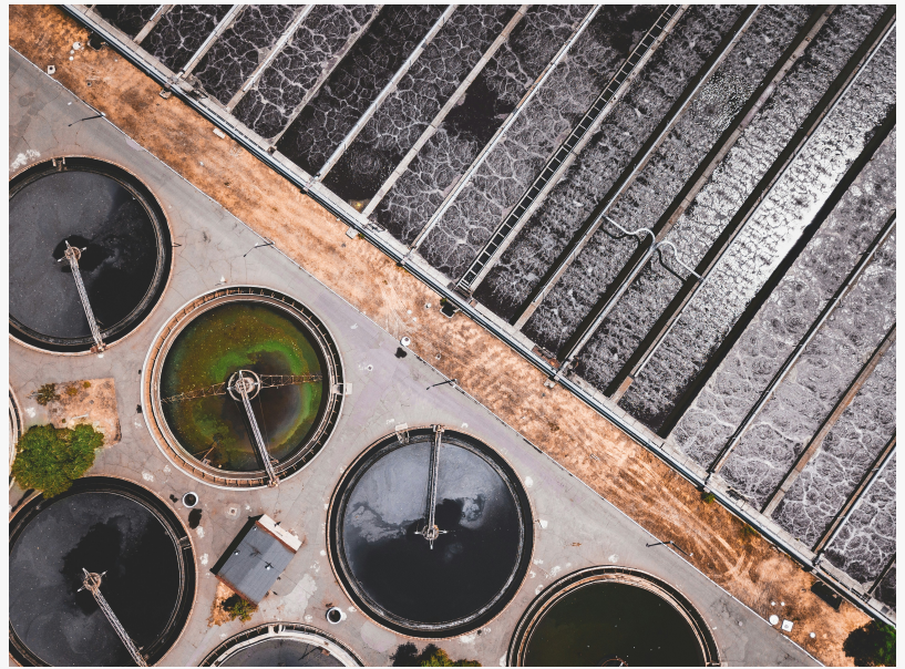
Sewage treatment facility
