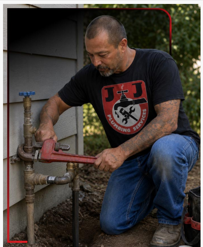
Natalio Pergis performing professional pipe repair and evaluation on an exterior water service line, helping homeowners address aging infrastructure in Kern County.
