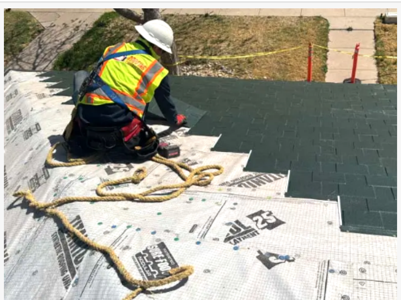
A professional roofing specialist installs new asphalt shingles during a residential roofing project in El Paso, highlighting the importance of proper installation and roof condition maintenance.
