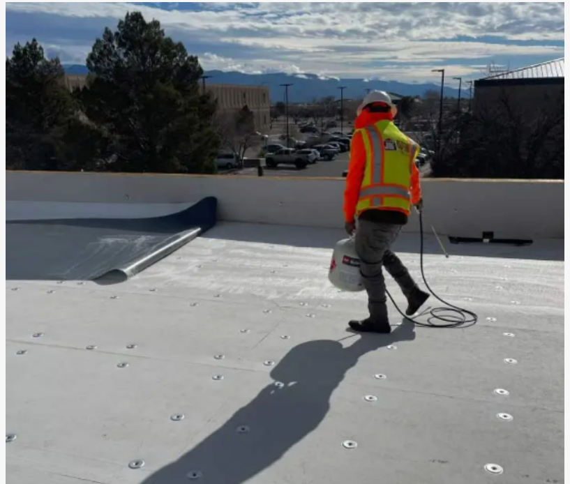
A JM Roofing and Construction technician applying commercial coating materials in El Paso, demonstrating high-quality systems that provide resistance and long-term durability.
