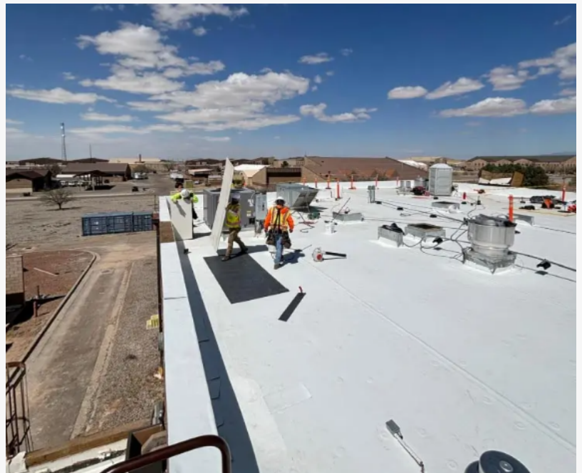
JM Roofing and Construction crews performing high-wind restoration and commercial TPO roofing work, illustrating the advanced roofing systems utilized across the El Paso region.
