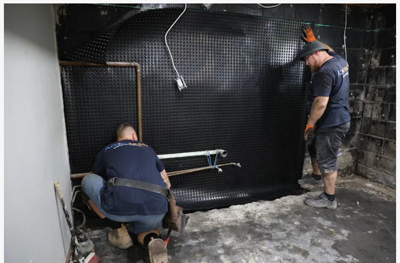
The Aquatech team completing another basement waterproofing repair job for an Ontario family.
